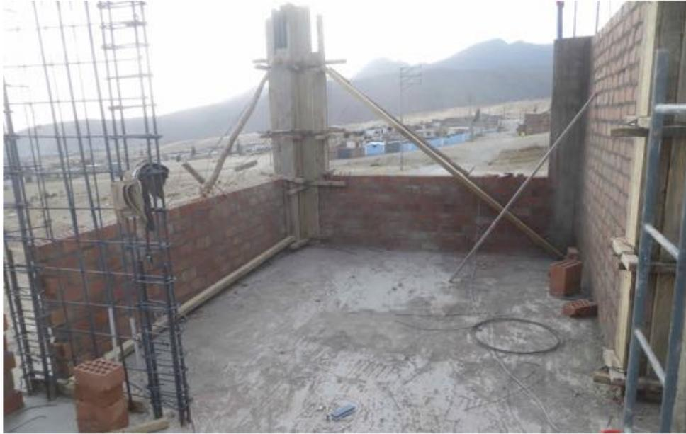
The roof has been poured over the first floor bathrooms and storeroom
