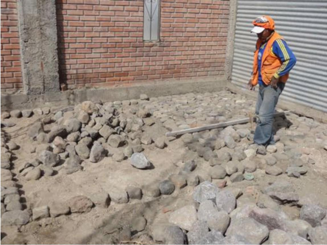
they're now getting ready to pour a concrete floor in that area and turn it into an expanded worship space. Experience has shown that this is the best way to do floors here in Arequipa. In case of an earthquake, the rocks under the concrete allow the earth to move underneath the building without cracking the concrete floor - one of many construction techniques they've learned here over centuries of experience living and building in a seismically active zone.
